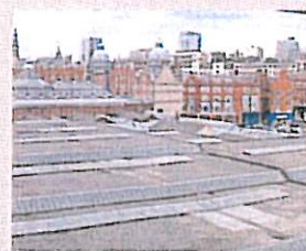
View of roof over covered market towards c1904 market hall
