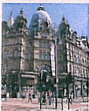
Corner entrance at New Market Street, Vicar Lane and Kirkgate
